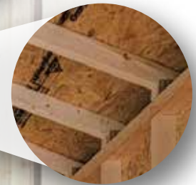
16" Roof Truss Framing
