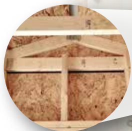
16" On-edge Gable End Framing
