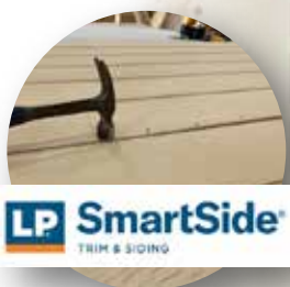
Hand-set Nails & LP Siding
